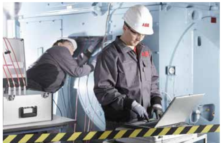
Condition monitoring technologies, including ABB LEAP (Life Expectancy Analysis Program) and PdMA MCEmax
