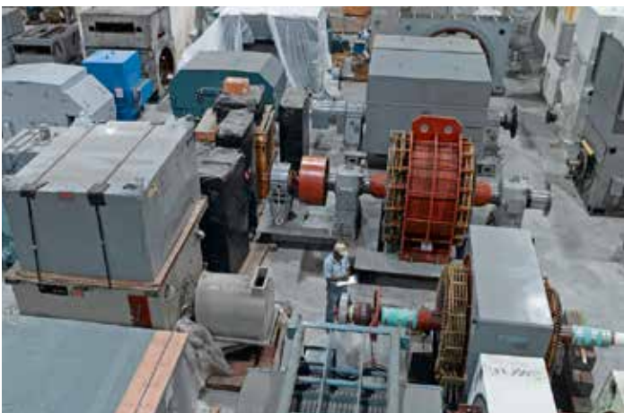
Over 300,000 square feet of dedicated warehouse space across North America, to store and maintain critical rotating assets
