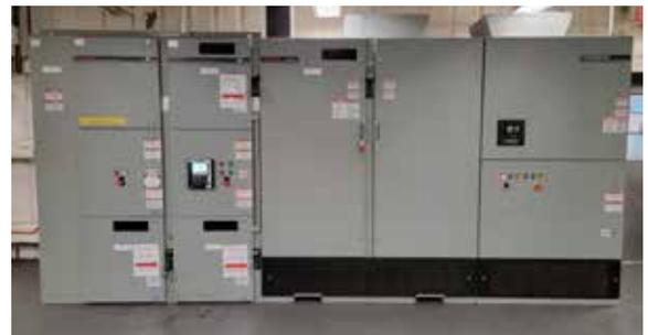
Toshiba T300MV2 VFD with Synchronous Transfer.
